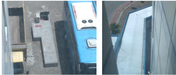
Waste water treatment plant
